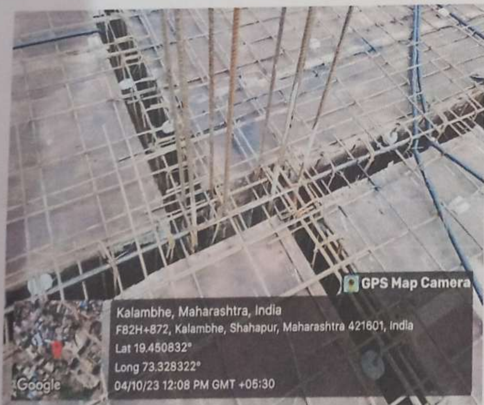
Beam Column Junction
