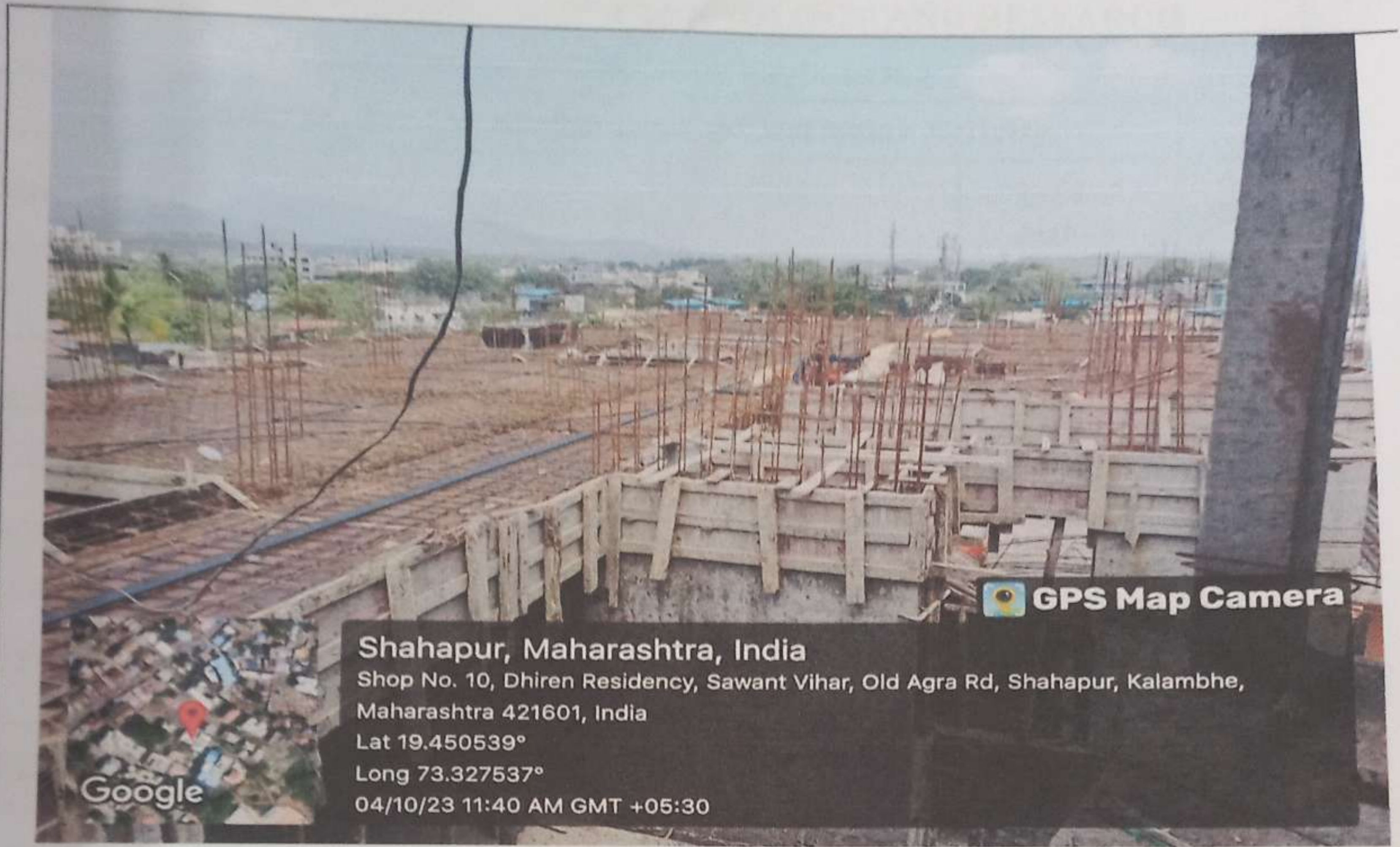
G+7 RCC frame structure Site View.
