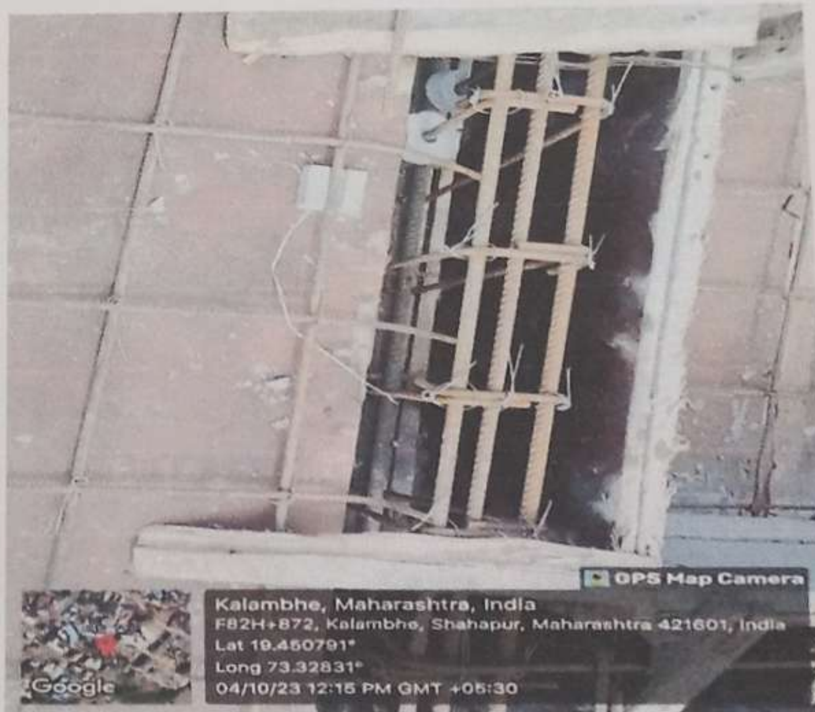
Beam Reinforcement detailing
